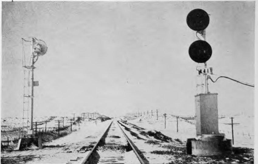
Intermediate signal with second unit to display the yellow-over-yellow aspect
