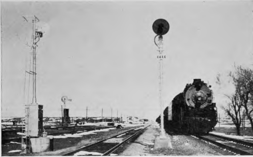
View showing train on the main track, and the intermediate automatic signals on the siding at Glazier
