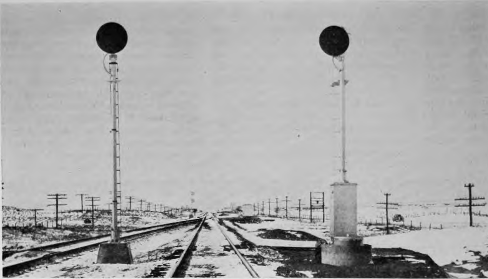
Above—Signal at left, for directing trains to leave a siding, is a high signal and located between siding and the main track.
