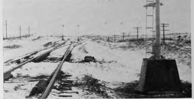
Above—Signal at left, for directing trains to leave a siding, is a high signal and located between siding and the main track.
