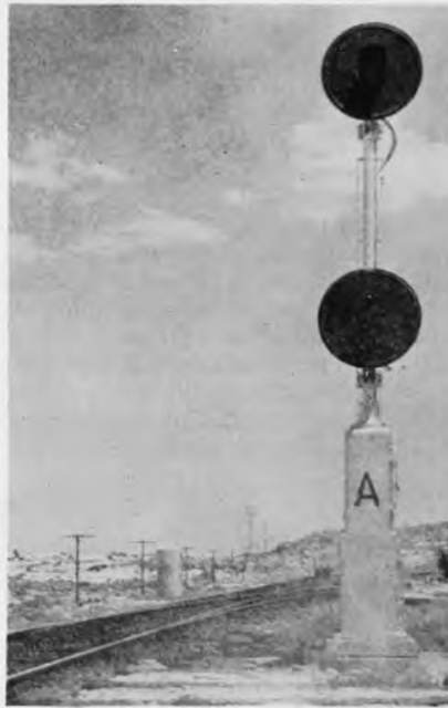
Signal at west end of Lakeside
