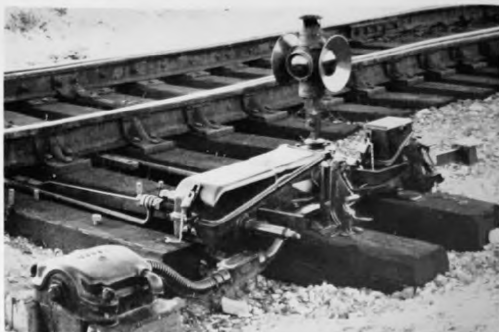
Hand-throw switch-and-lock machine with electric lock on the lever
