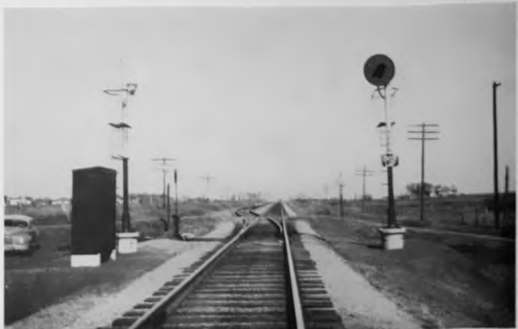
Signals at end of siding in single-track automatic block territory in Texas
