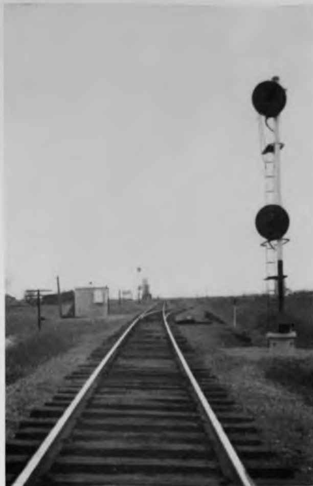
Signals at a typical power-siding switch in single-track C.T.C. territory
