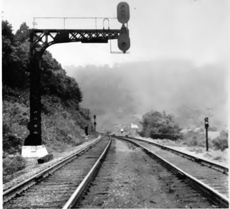
Signals at the spring switch at the west end of Wagner siding
