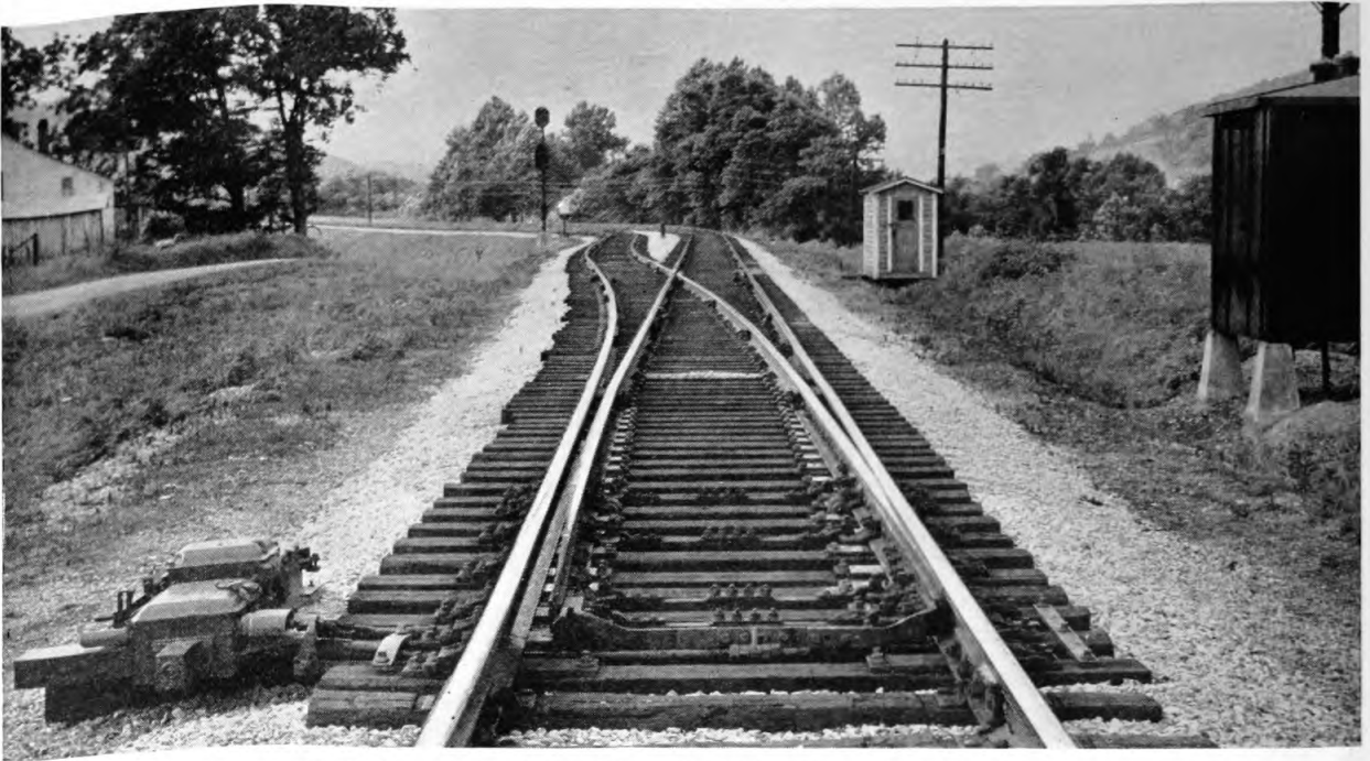
Typical power switch layout on centralized traffic control territory
