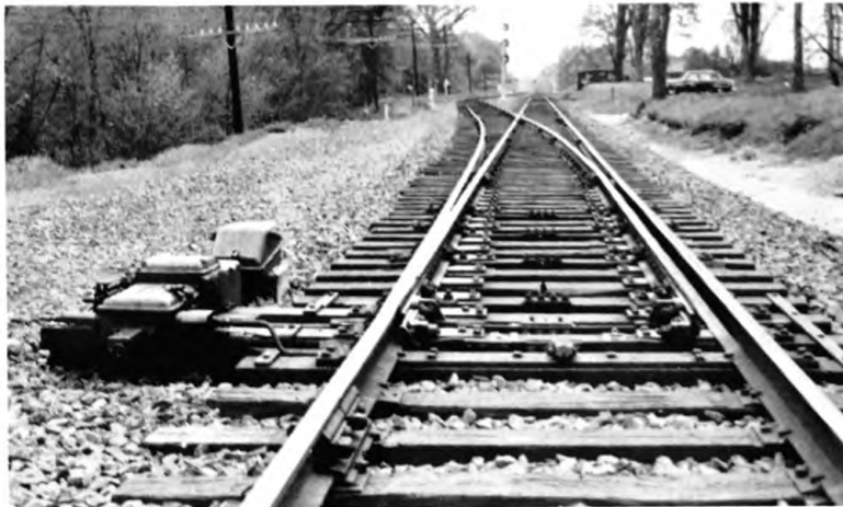
Power switch machines are used at the ends of the sidings
