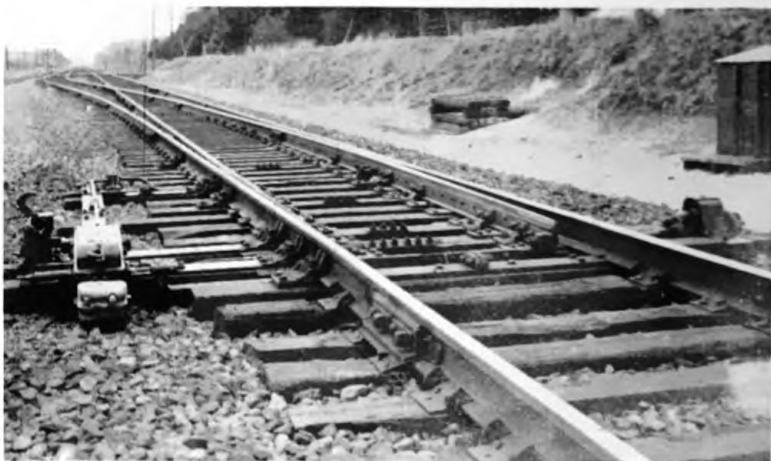
Spring switches are used at the ends of double track
