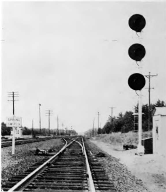
Signals at end of double track
