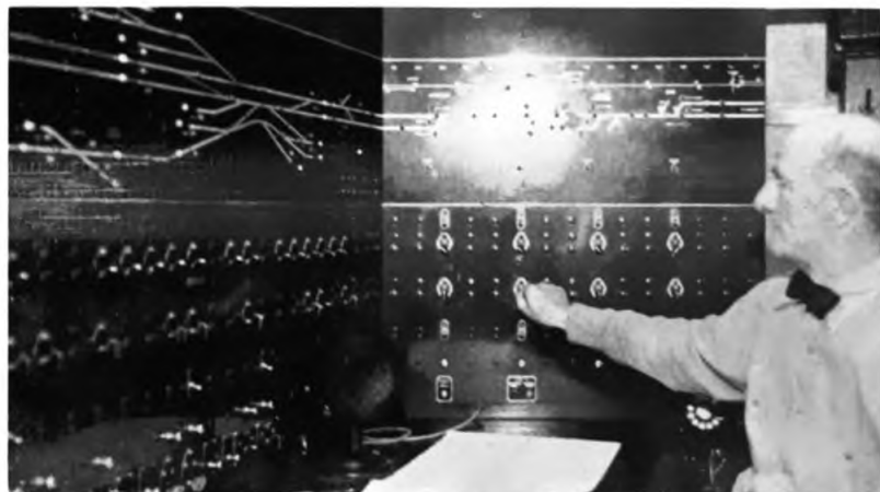
This right wing panel controls the new Amoskeag-Concord section
