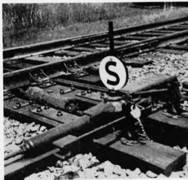
Each spring switch layout includes a hand-throw mechanism with an oil buffer and spring
