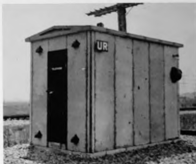
Pre-cast concrete sectional type of house for relays and battery at UR
