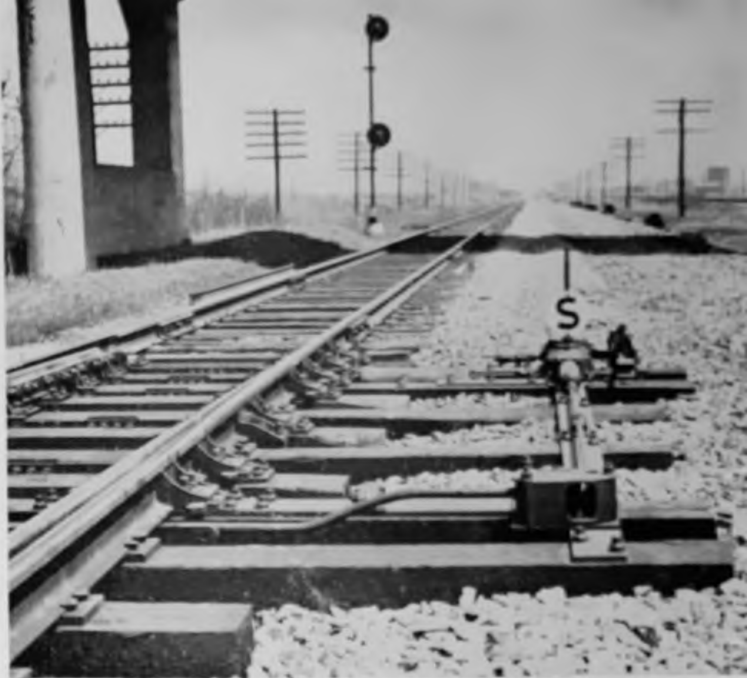
Signals and switch at end of double track at UR
