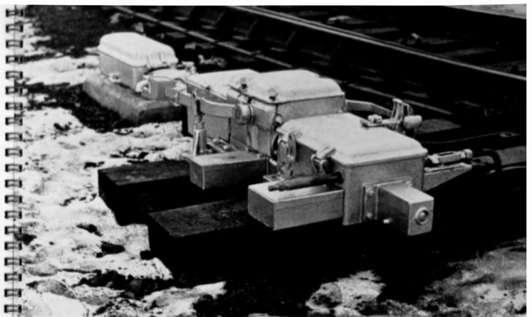
DUAL CONTROL electric switch and lock movement.
