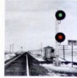
Switch operates—signal clears
