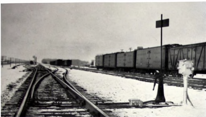
LOOKING WEST from electric switch lock installation at Brush.
