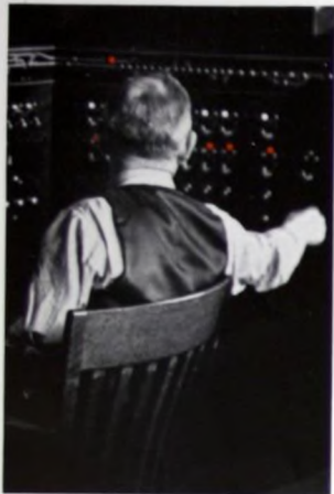
DISPATCHER lines up switches for main line and clears westward signals.
