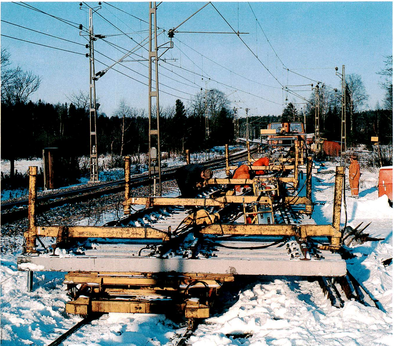
Turnout exchanger being used to lay prefabricated point
