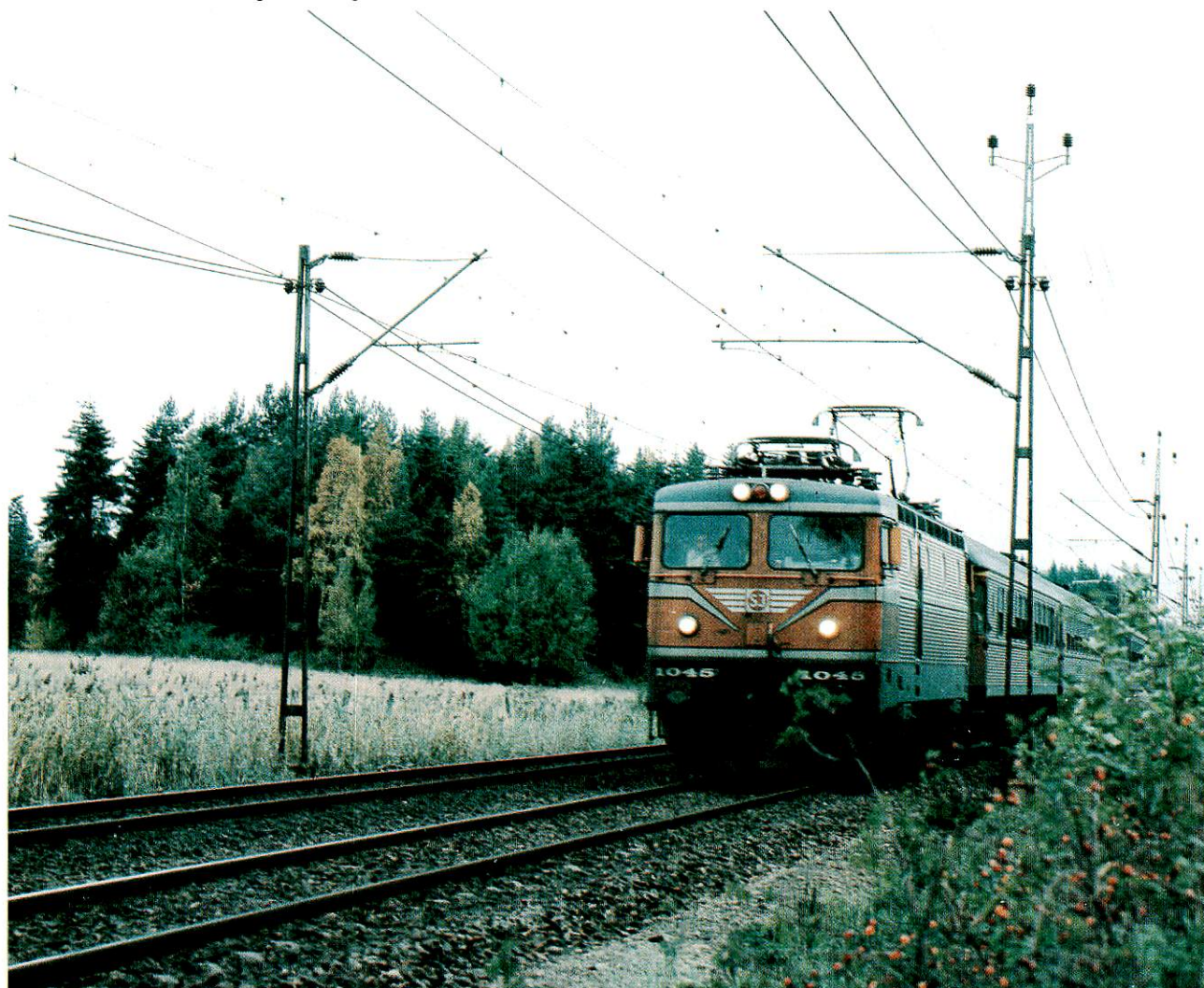
Overhead contact lines designed for high-speed trains
