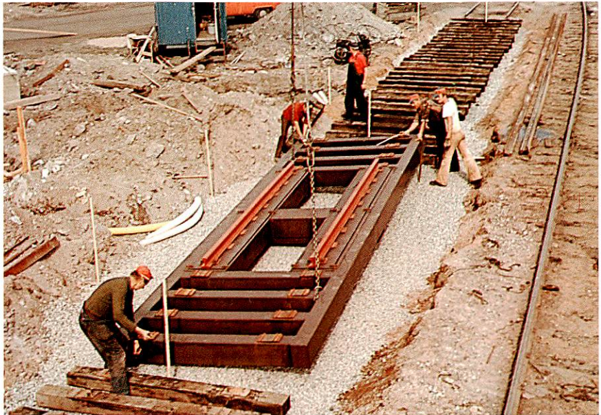
Electronic scale during installation
