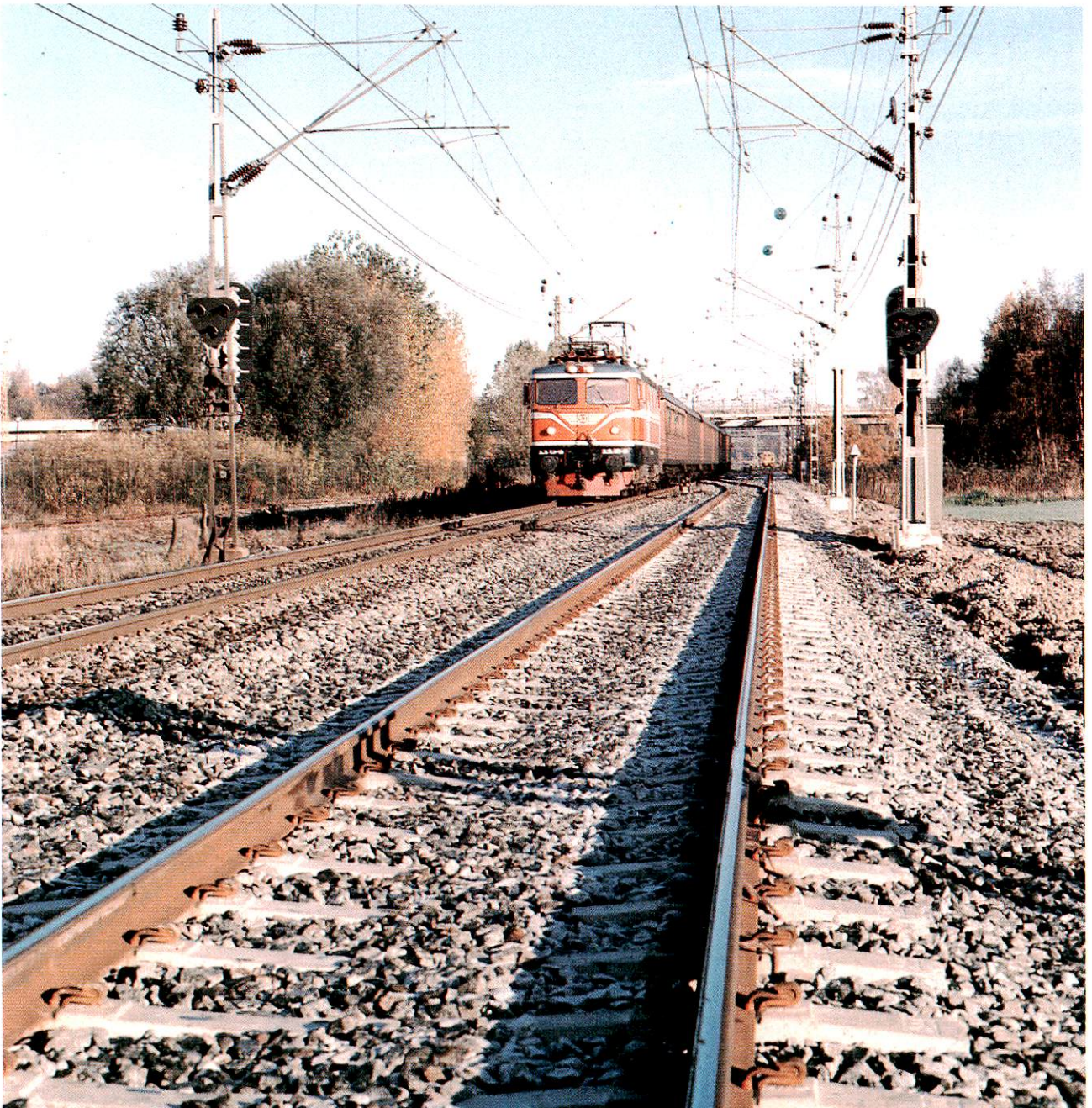
Double track with concrete sleepers
